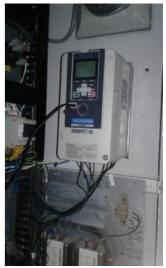
• New cable for Y271 (InvDp) from S3 and S4 (link), connect Output channel 5 on 2nd Output slice (labelled 5)
