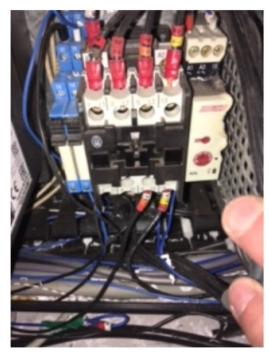
The timer and contactor were added 15 years ago on flowlines when the old DOS PC used to have a boot-up problem due to the drives switching on at the same time as the PC power supply, causing a power drain.
